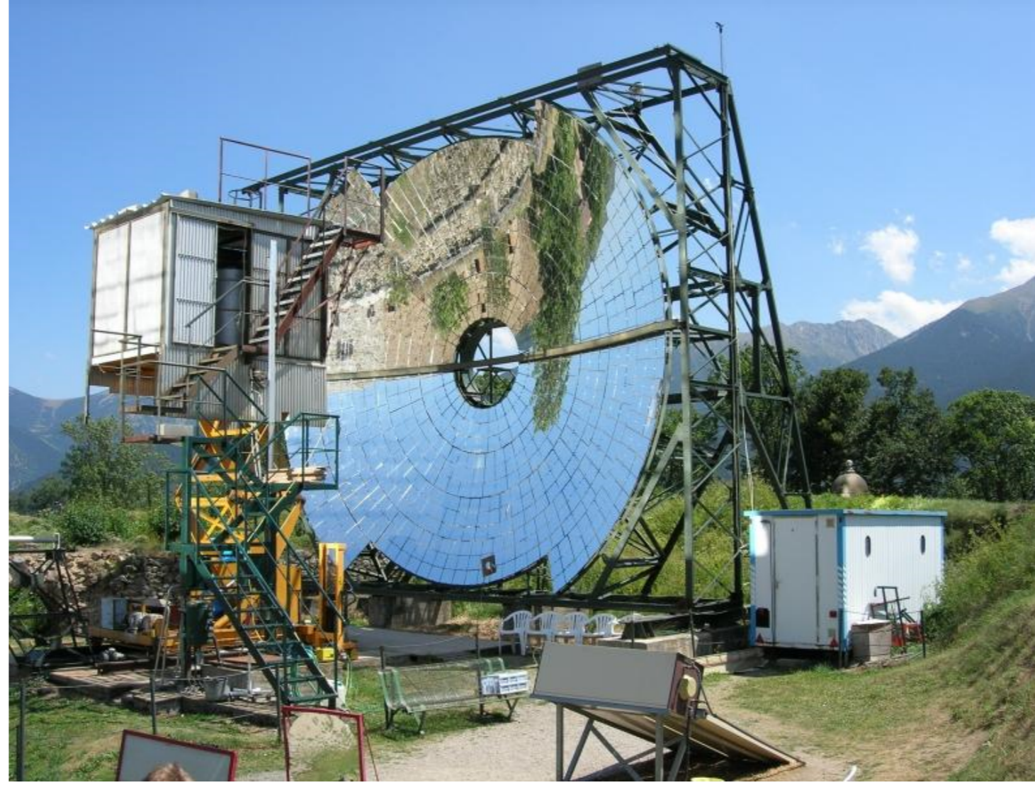
Parabolic mirror of solar oven in Mont-Louis
